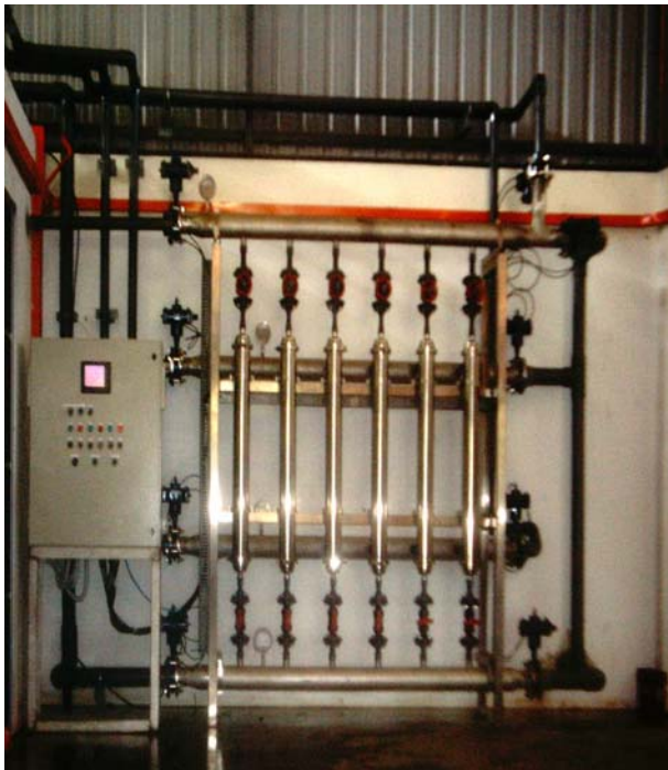
Membrane Filtration Using Ultra-pore size- 0.1-0.01 \mu for removal of bacteria, heavy metals and suspended solids.
